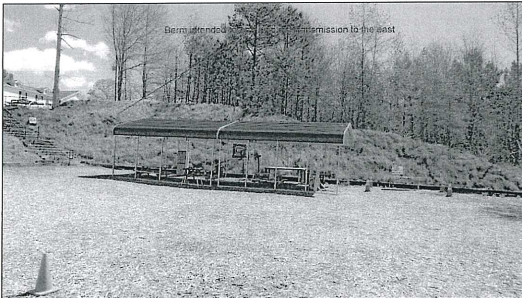
Photo #5 Sound abatement berm behind the ready area on the pistol range.
