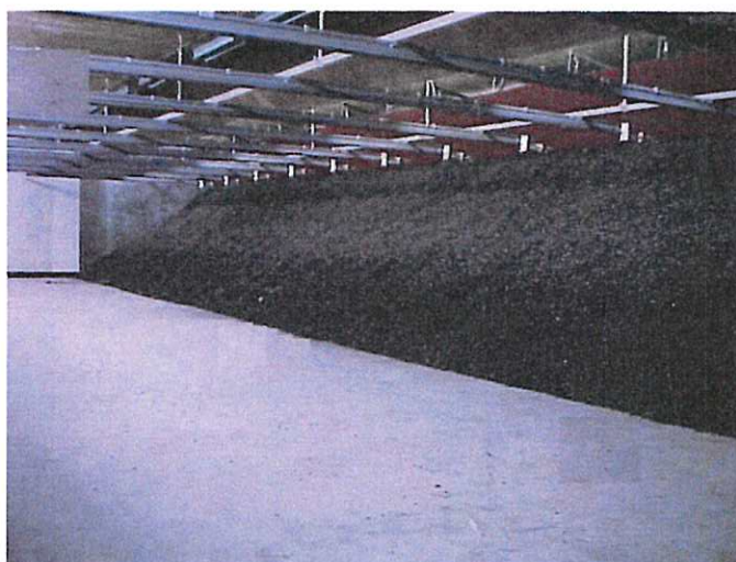
Figure 7 Rubber bullet trap
